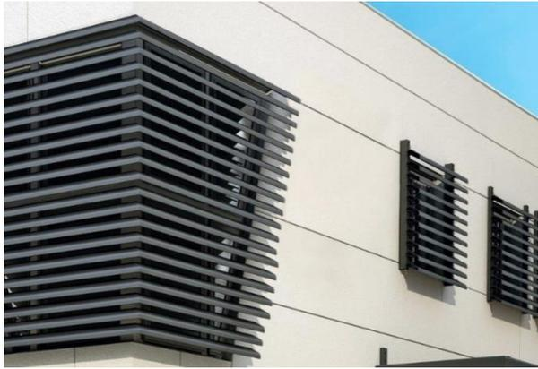
Figure III.74 : Lames brise soleils en aluminium. Source : [http://www.alluco.com/prods/Brises\\_Soleil/Brise\\_Soleil\\_Vertical](http://www.alluco.com/prods/Brises_Soleil/Brise_Soleil_Vertical)
