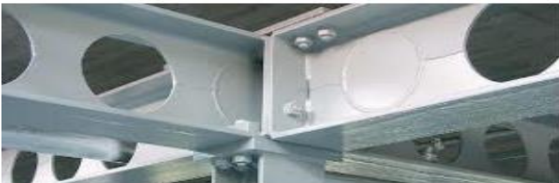
Figure 69: fixation poteau-poutre (source: google image)
