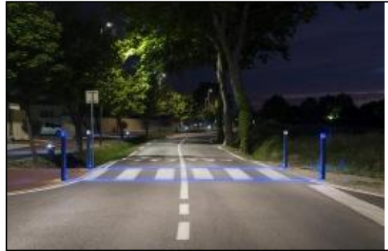
Figure92: lampadaire infrarouge Source :Google image
