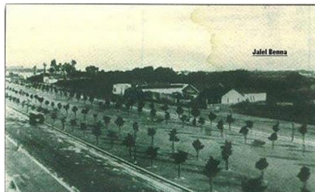
Figure 36: Ancienne photo de l'avenue Habib Bourguiba Source : https://www.pinterest.com/pin/717901996821503087/visual-search
