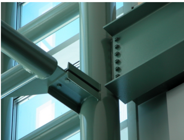
Figure 114 Steel colomns and beams /source : tboake.com
