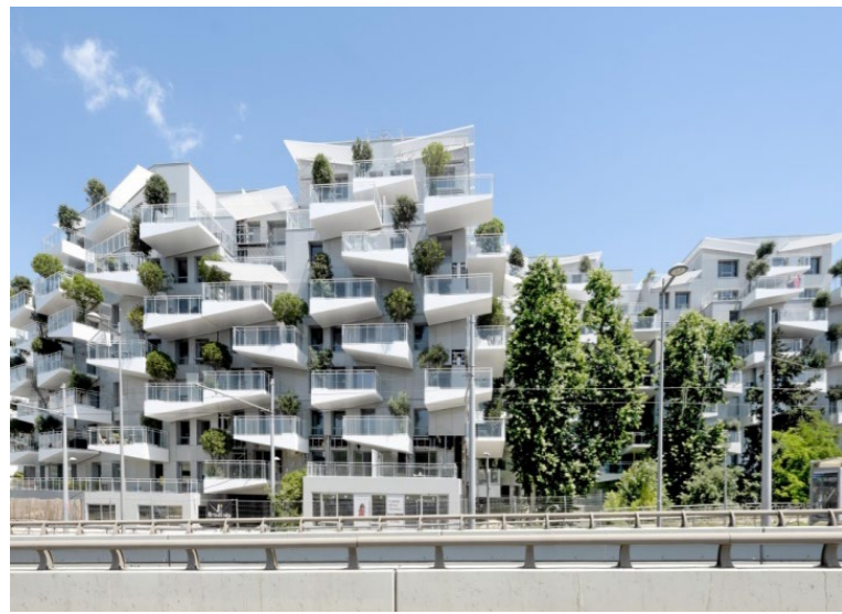
Figure 15 Prado Concorde apartments/ source: ArchDaily.com
