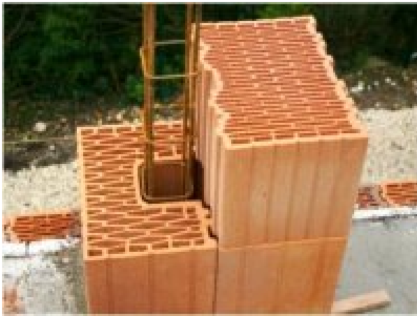
Figure 119 Monomur bricks/source:maconnerie.bilp.fr
