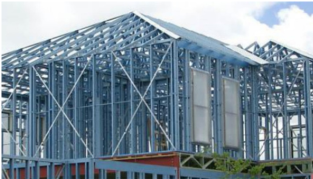
Figure 113 Metal structure/source: northern-weldarc.com
