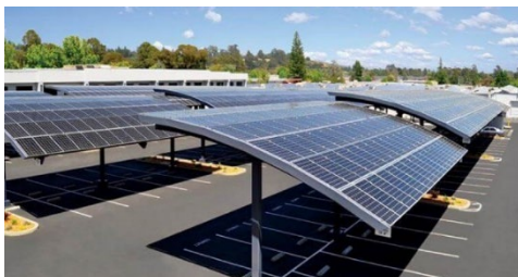
Figure 124 Solar panel parking roof /source: .indiamart.com
