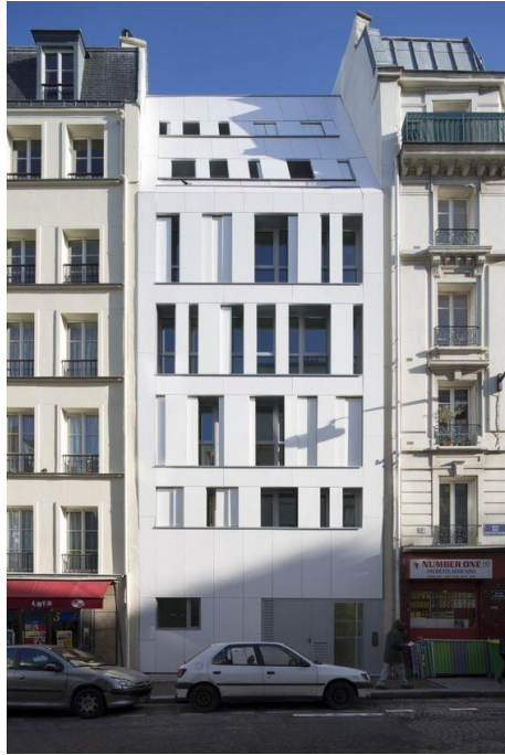
Figure IV-43 : Appartement 18th arrondissement of Paris, Paris, France
