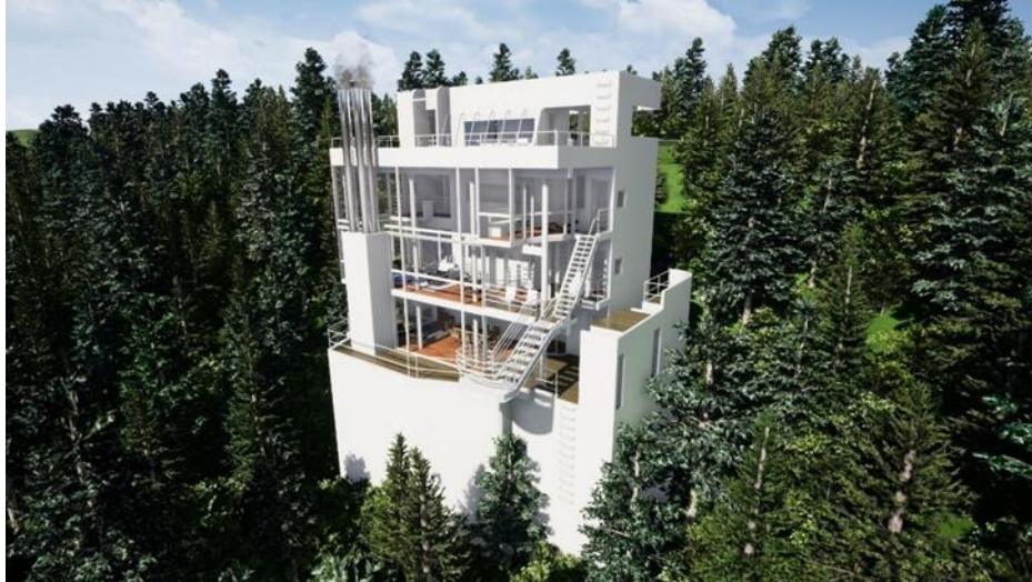
Figure 74: Richard Meier Douglas house an architectural masterpiece
