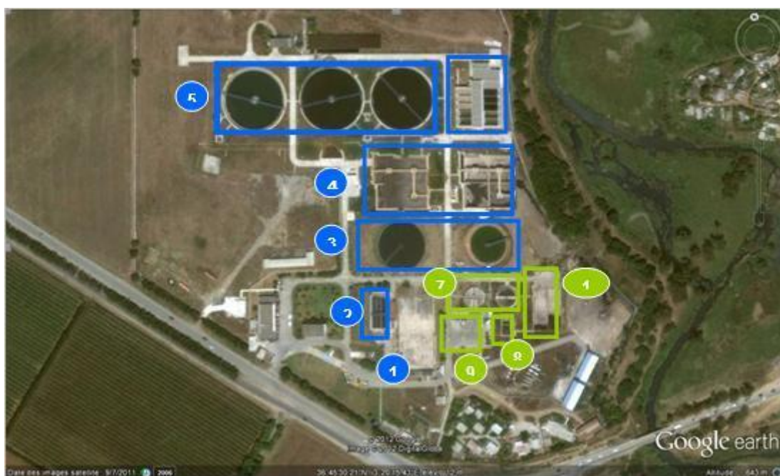
Figure 1. 5: Description et installation de la STEP.[1]
