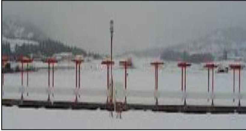
Figure 1.3: Antenne Localizer
