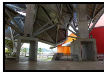
Figure 2-4 Atrium centrale Source: visitpanama.com
