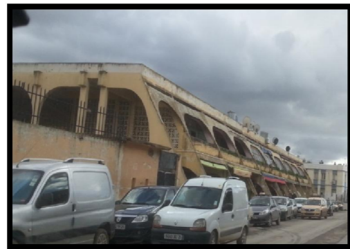
Figure 3.171: La façade principale
