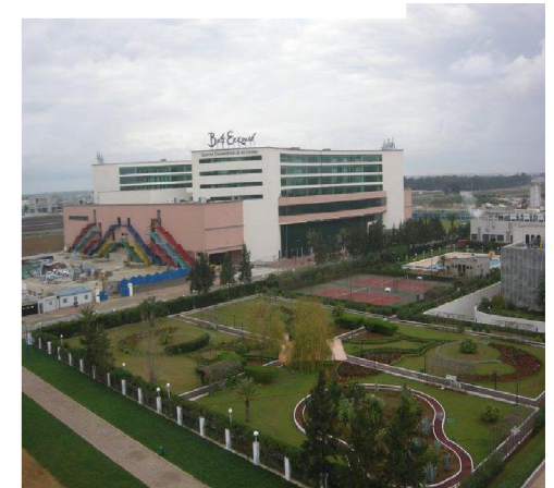
Figure 3.172: Centre commercial de BAB Ezzouar
