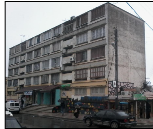
Figure 29 : La façade principale
