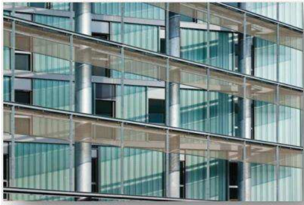
Figure 21 : BRISE SOLEIL, FAÇADE SUD
