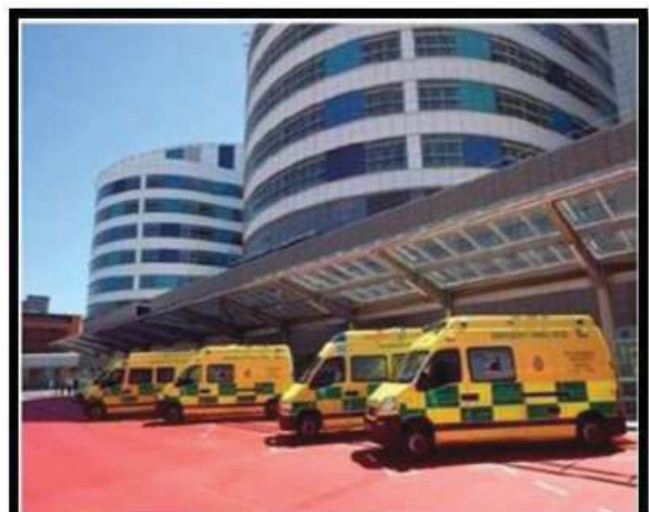
Figure 34 : ENTREE DES URGENCES DE L'HOPITAL QUEEN ELIZABETH Source : www.designbuild-network.com
