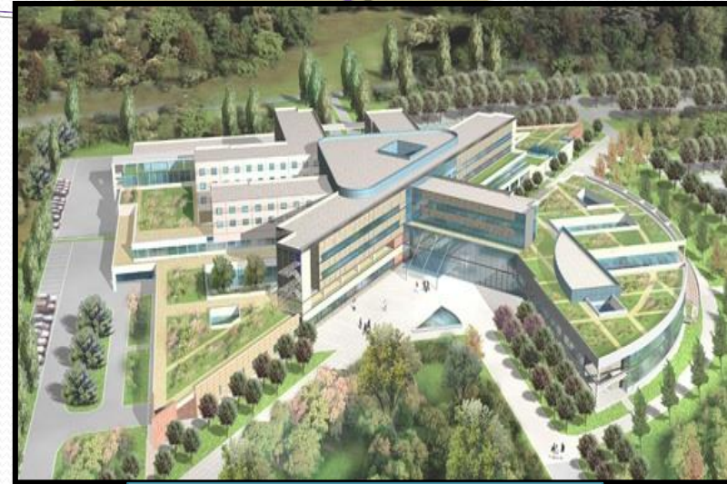
Hôpital Saint Dizier – France
