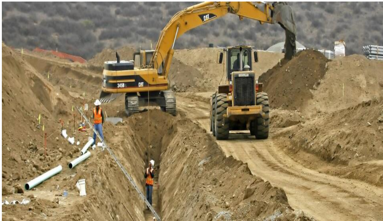
Figure 4.1. A deep trench at residential construction site [40].
