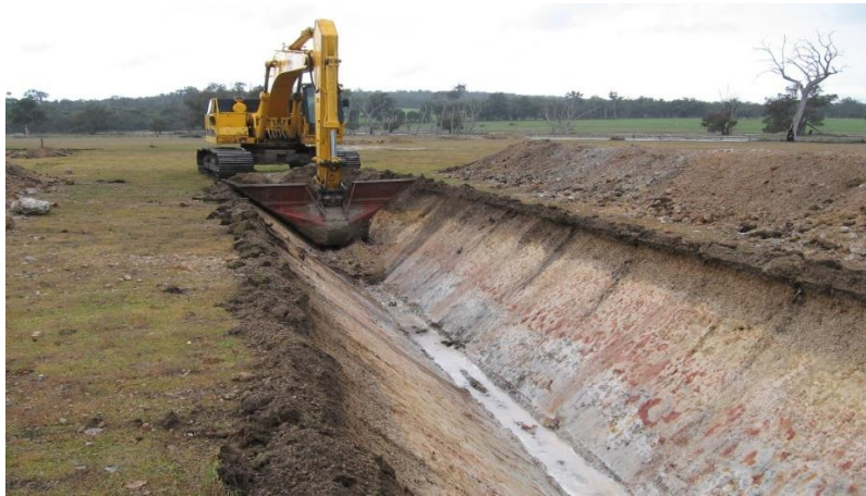
Figure 2.11: V- shaped infilled trench [33].
