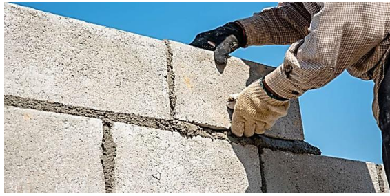
Figure 1.13: Mortar laying [23].
