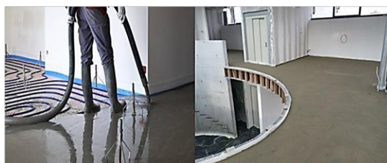
Figure 1.15: Fluid screeds and cement screed [23].
