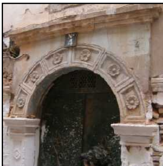
Figure II.3: Chambranle en tuf
