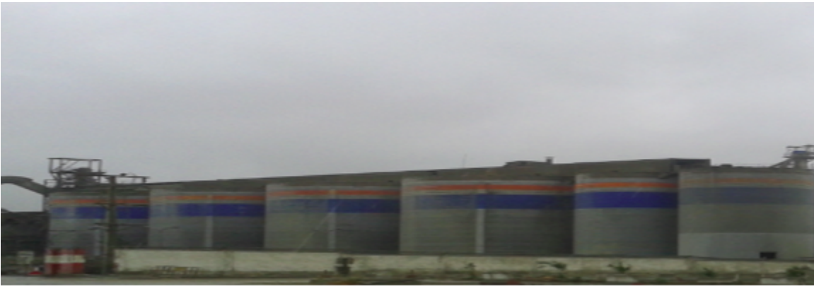
Figure I.17: Silos stockage de clinker.
