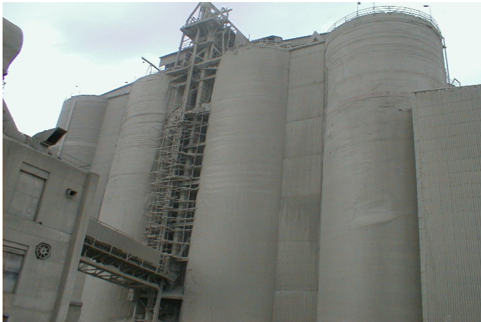
Figure I.19: image silos de stockage du gypse, calcaire, ciment.
