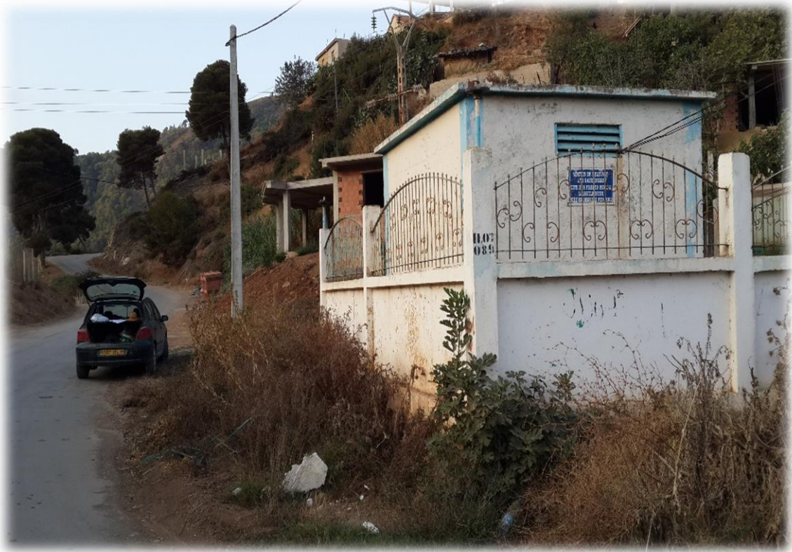
Figure III.2 : Poste de relevage.
