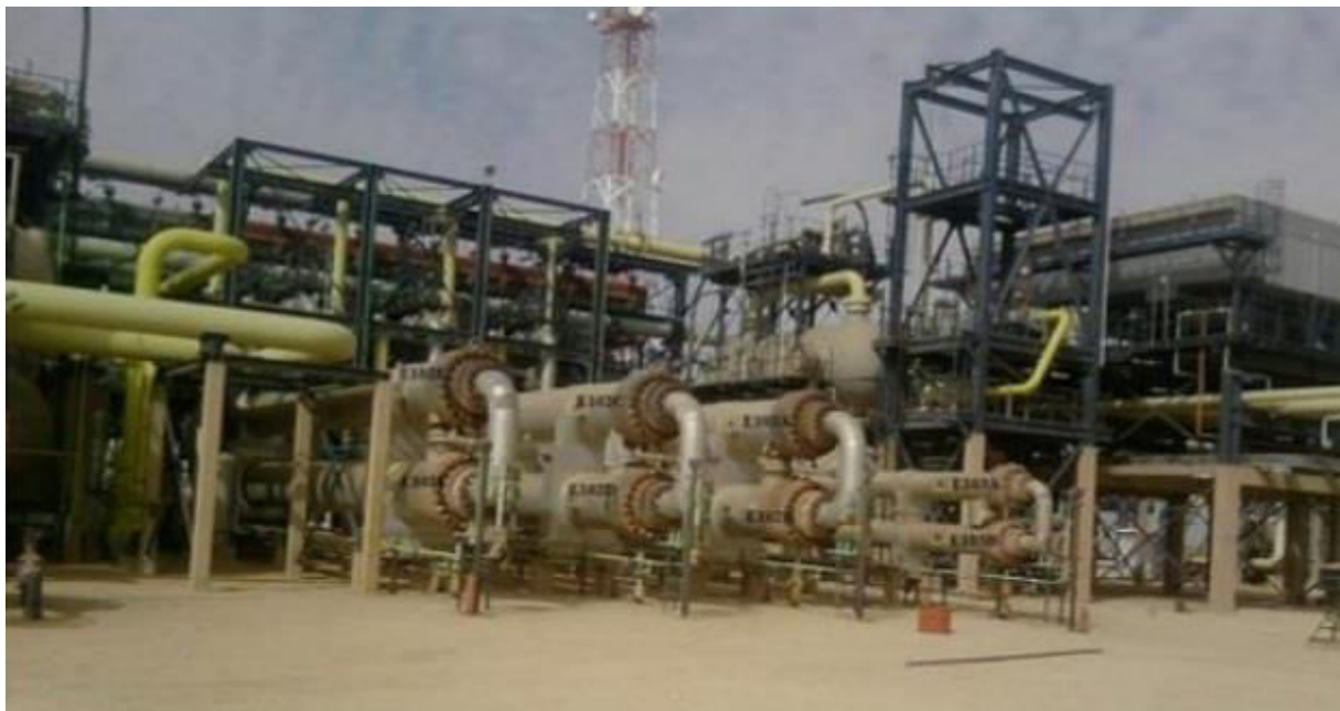
Figure.3.16 Countercurrent exchangers (high pressure part) E102 A/B/C/D/E/F+E103A/B
