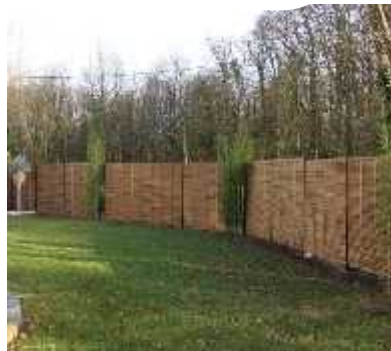
Figure 66: palissade traditionnelle en bois (source: http://www.achievenewsfrance.tk/images/Palissade%20traditionnelle%20en%20bois )
