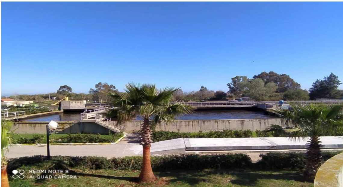
Figure 2.1: La station d'épuration de CHENOUA
