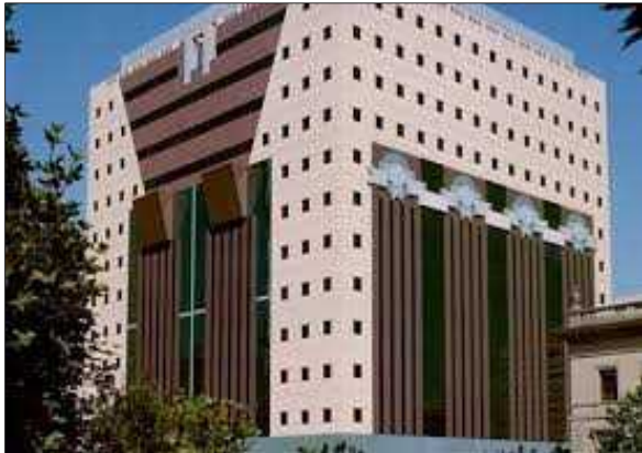
Figure 3.29 : Public Services Building (Portland, 1982) Michael Graves
