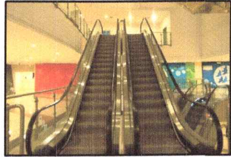
Figure 3. 44 : Escalator Source : Google image
