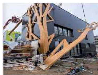
Figure 110 :chantier de chaville
