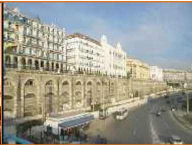
Fig 06 : Architecture colonial . Source : Google image
