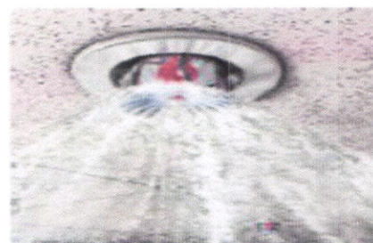
figure N°115 :sprinklers
