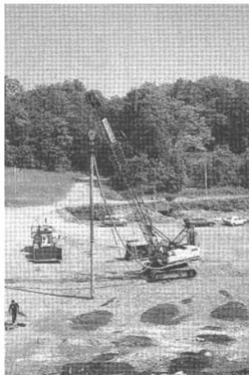
Figure I.8 : Chantier de vibrocompactage. [7]
