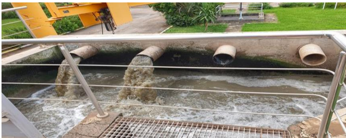
Figure 2.5: poste de relevage.
