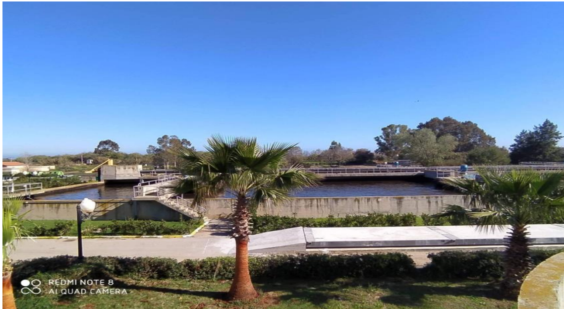
Figure 2.1: La station d'épuration de CHENOUA
