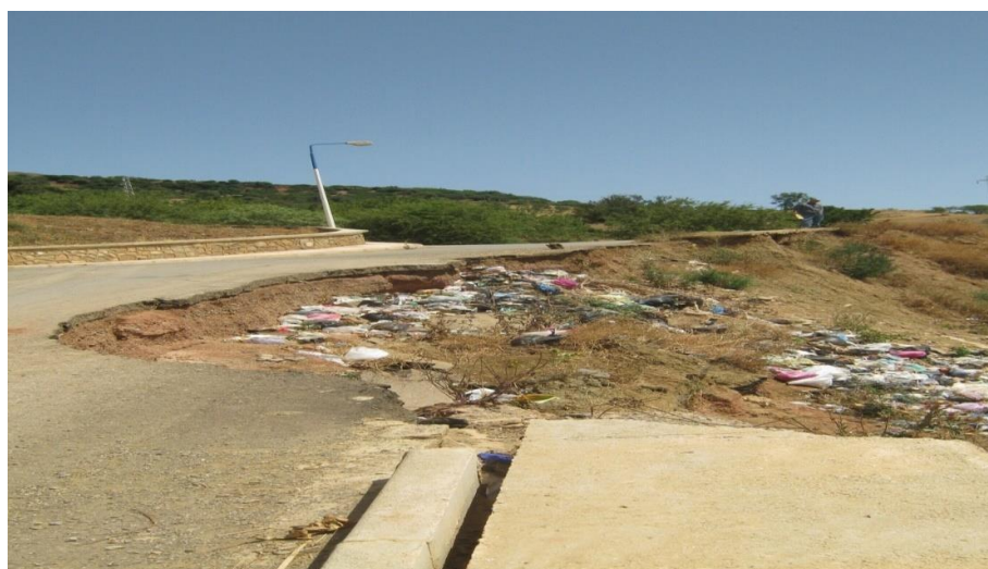
Figure II.6: Photo de la niche d'arrachement
