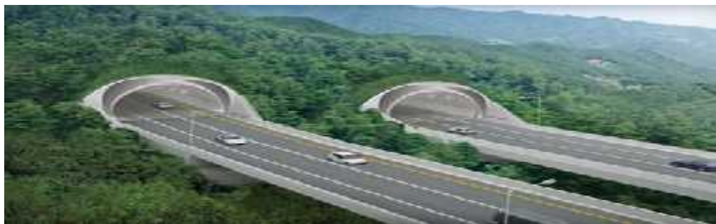
Figure II-11 tunnel de Texenna. Source : http://www.jijel.info
