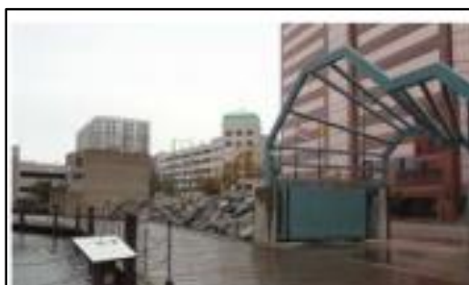
Figure 73. Installation d'écluse source : www.norfolk/city.com
