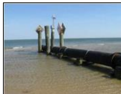
Figure 72. installation d'exutoires source : www.norfolk/city.com
