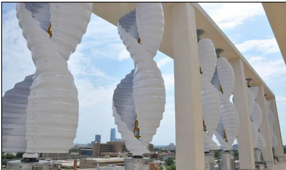
Figure 33. Intégration de l'énergie du vent dans la construction. Oklahoma Medical Research Foundation-USA source: www.treehugger.com/renewable-energy/largest-building-integrated-wind-power
