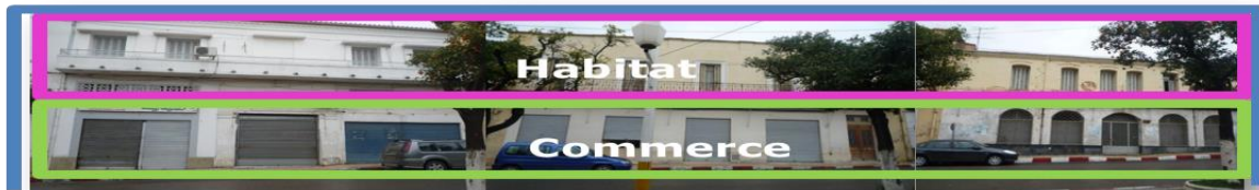
Figure 100: La façade urbaine.
