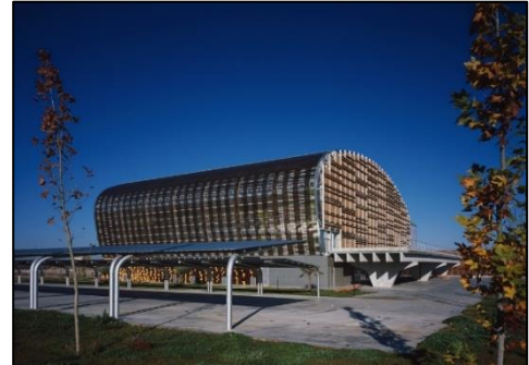
Figure I-71 : Telefonica Moviles (source: Google image )
