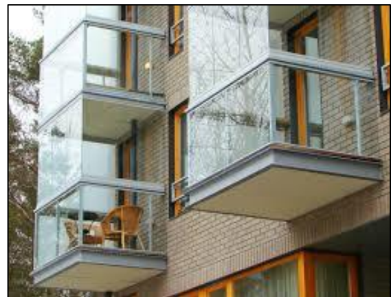
Figure I-25: la loggia vitrée source ( Google image )
