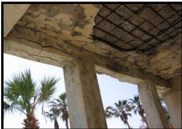
Concrete corrosion
