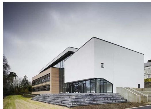
Figure 94: Photo du projet; Source : ArchDaily.
