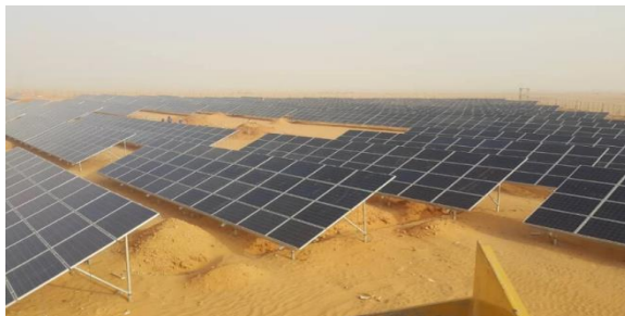
Figure 1.7 : Photovoltaic power plant with a capacity of 5 MW in Reggane, Adrar [9].
