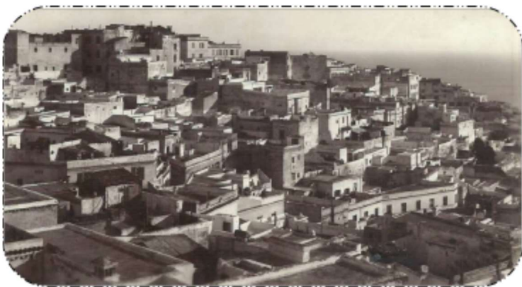
Figure 1-13: Photo de la Casbah d'Alger. Source : http://www.algermilitaria.com/pages/la-casbah/la-casbah-histoire-et-culture/la-casbah-d-alger.html .
