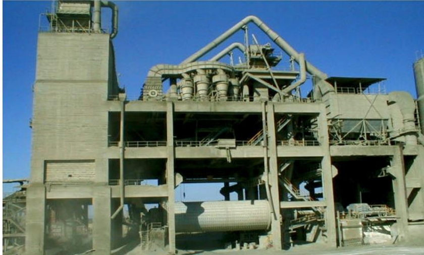
Figure 1.2 : Atelier broyage ciment
