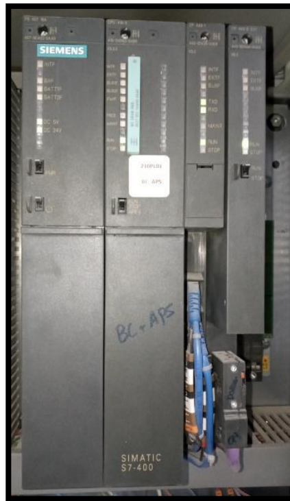
Figure 3.3 : L'automate S7-400
