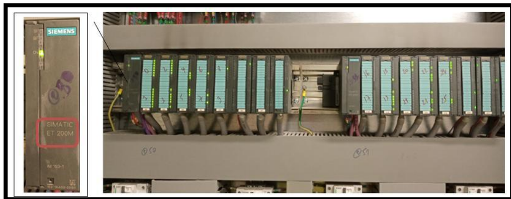
Figure 3.3 : L'automate S7-400
