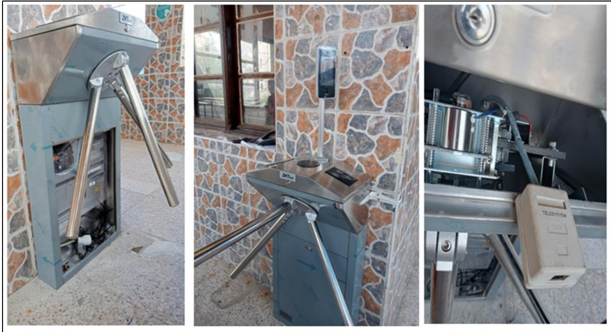
Figure 4.9: The installation of turnstiles with the V5L.
