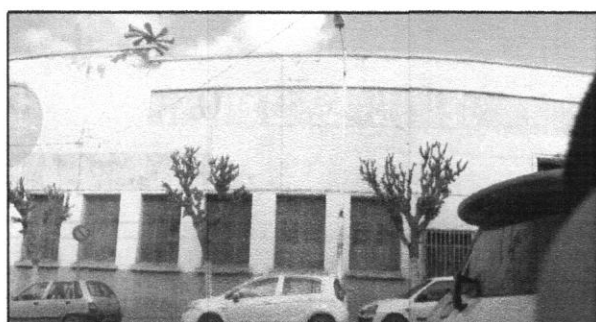
FIG 20.20.03:Façade de C.E.M.
