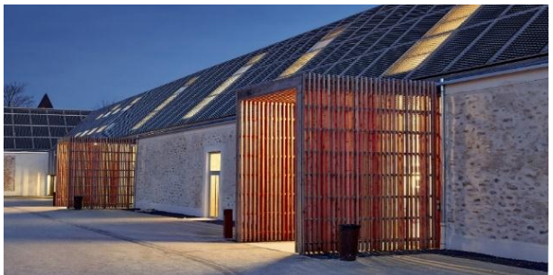
Figure 38 : Photo montrant l'ambiance lumineuse. Source : Arch Daily.
