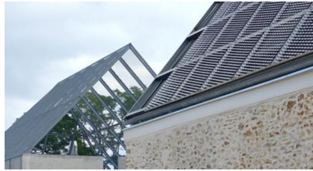
Figure 37 : Photo montrant la nouvelle charpente. Source : Arch Daily.
