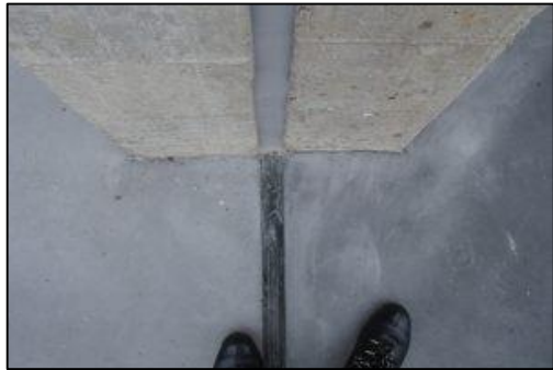
Figure 96: joint de dilatation.
