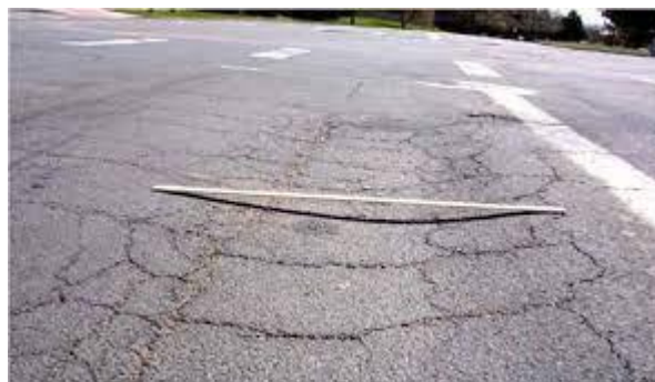
Figure I.18: Rutting [5]
