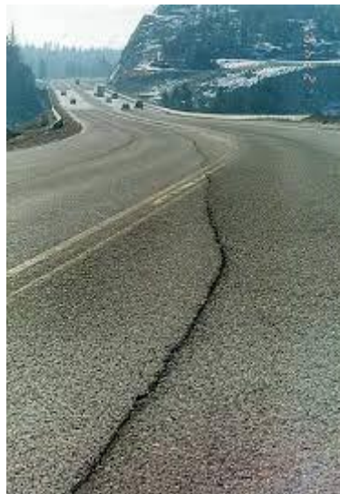
Figure I.14: Longitudinal Cracking [1]
