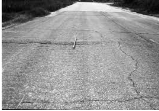
Figure I.21: Upheaval [5]
