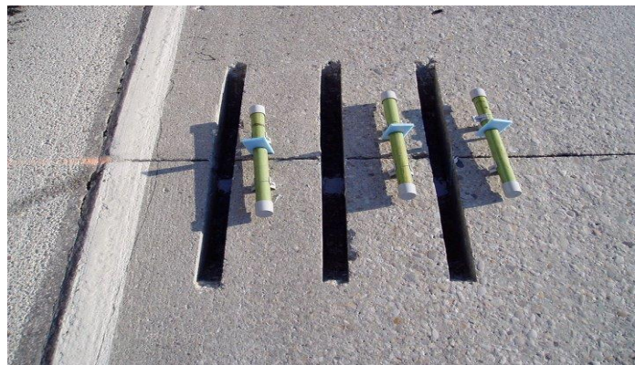
Figure I.34: Dowel Bar Retrofit [2]
