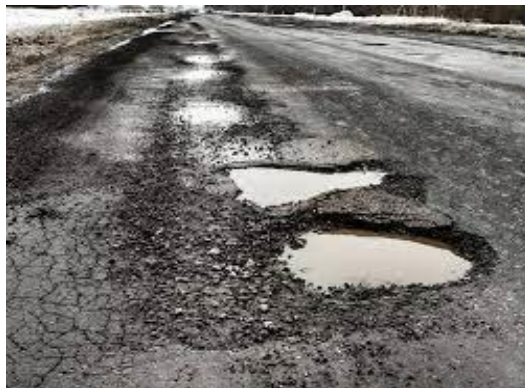
Figure I.24: Potholes [5]
