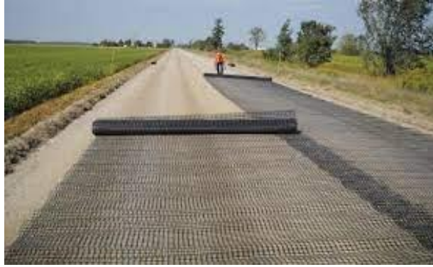
Figure I.31: Application of geosynthetic in the road repair [2]
