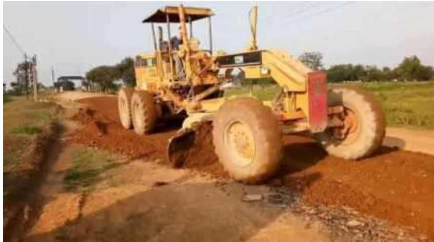
Figure I. 9: Laying Sub-base course [1]
