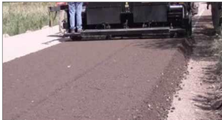
Figure I.3: Providing Base Course [1]
