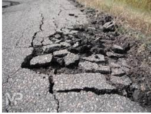
Figure I.13: Edge Cracking [1]
