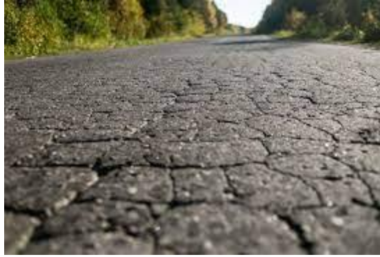
Figure I.11: Fatigue Cracking [1]
