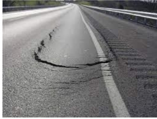
Figure I.17: Slippage Cracking [1]
