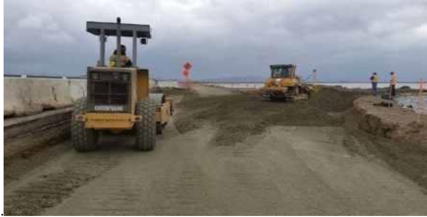
Figure I.4: Laying of Subbase Course [1]
