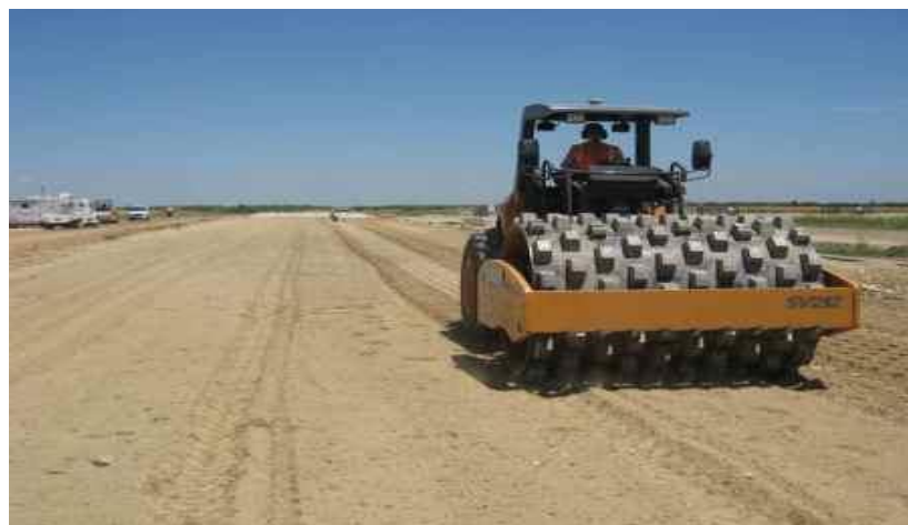
Figure I.10: Compacting Sub-grade [1]
