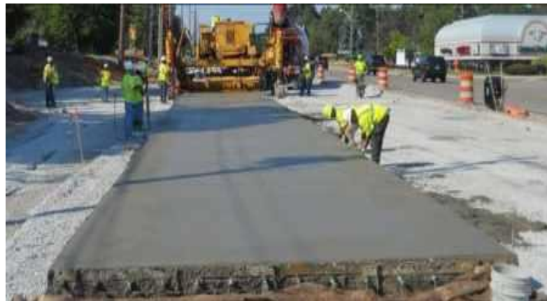
Figure I.2: Concrete Slab Laying [1]
