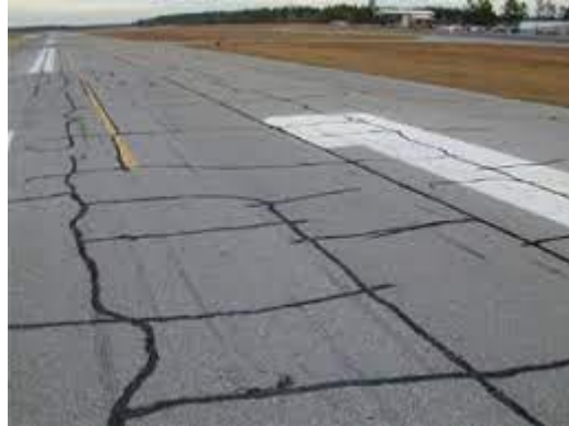
Figure I.12: Block Cracking [1]
