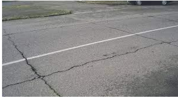
Figure I.15: Transverse Cracking [1]
