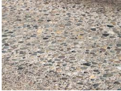
Figure I.25: Polished Aggregate [5]
