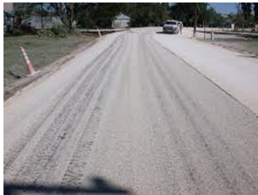
Figure I.29: Streaking [5]
