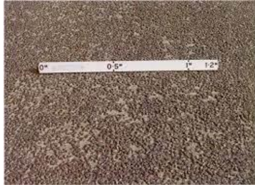
Figure I.28: Loss of Cover Aggregate [5]
