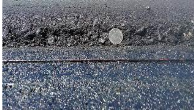
Figure I.33: Thin-lift asphalt overlay [2]
