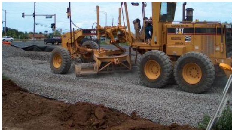
Figure I.8: Laying Base Course [1]
