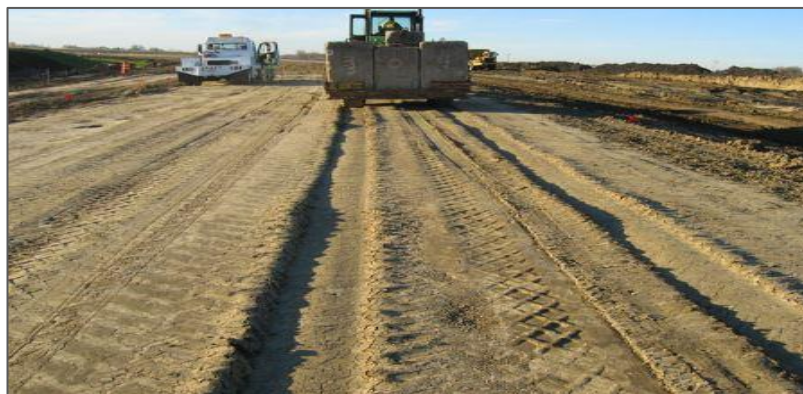
Figure I.5: Preparing Subgrade Soil [1]
