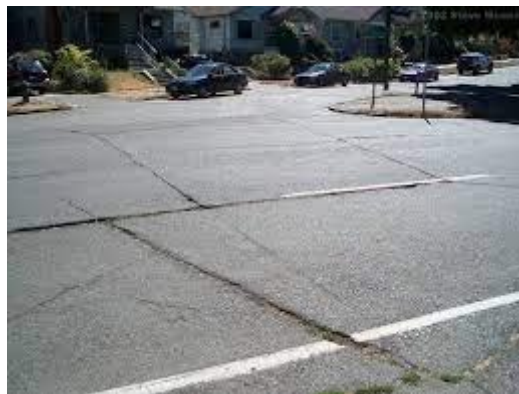
Figure I.16: Reflection Cracking [1]
