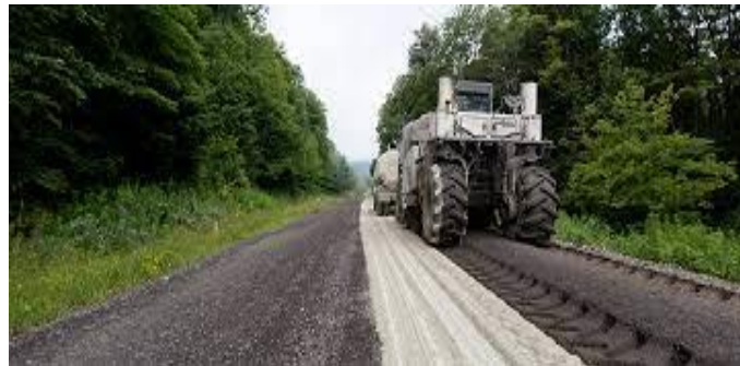
Figure I.32: Full-Depth Reclamation [2]
