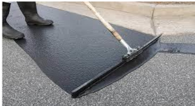
Figure I.30: Sealcoating [2]
