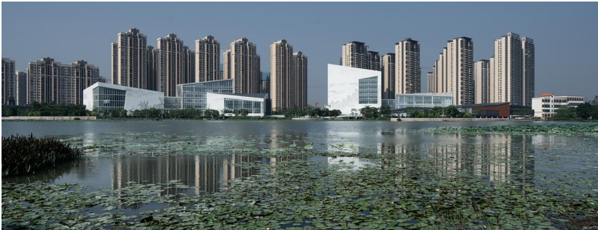
Figure 17: View from across the lotus pond. Image © Qingshan Wu
