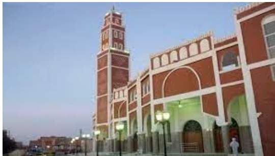
Figure 11: mosquée Mohammed Belkebir a adrar. Source : https://web.facebook.com/sedjad01/posts/33095957250208/
