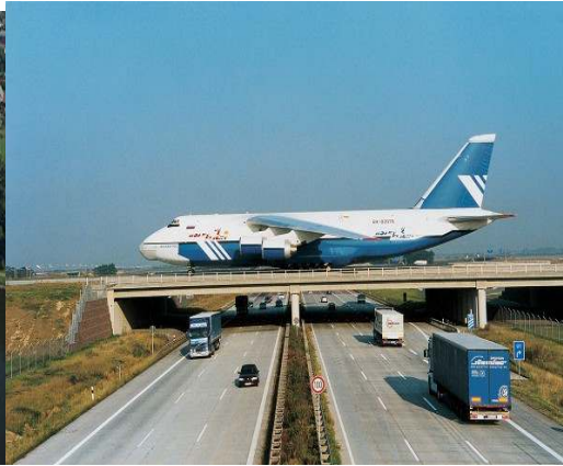
Figure I.4 Pont supportant un avion
