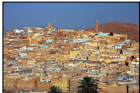
Figure 124: photo de ksar beni isguen. Source: OPVM
