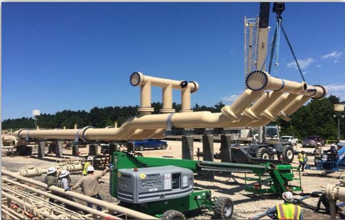
Figure II-26 : Slug Catcher [8]
