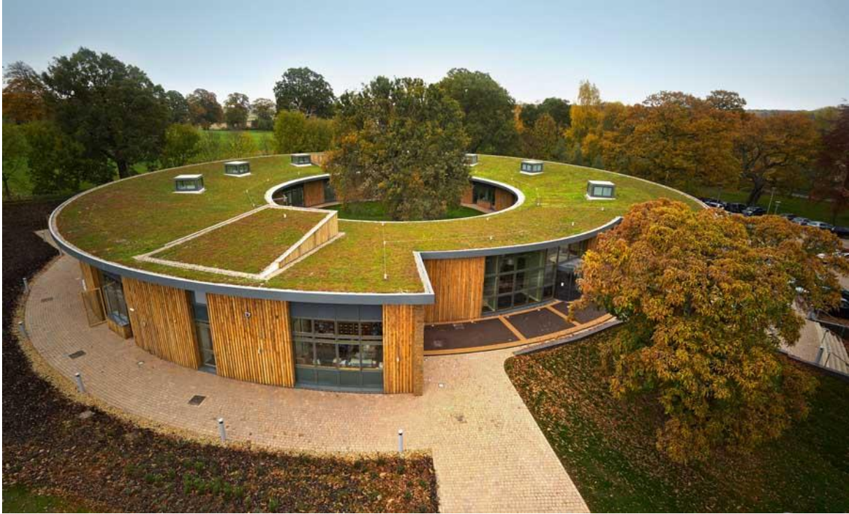
Figure 9 Green roof – Wikipedia [56]
